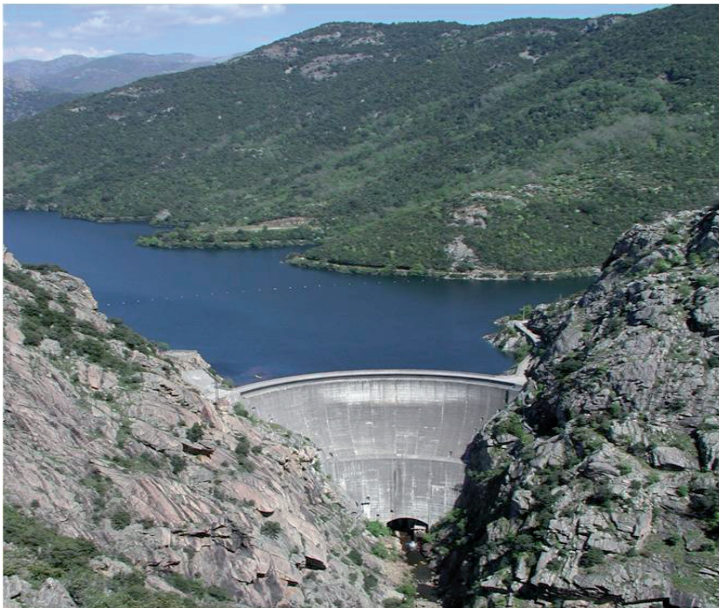
Corsica: Tolla dam - Hydroelectricity and water supply for Ajaccio and its region (South of Corsica). Built on the Prunelli river in 1960 by EDF, the Tolla dam which contains 31 Mm 3 is used for water supply, irrigation and production of hydroelectric energy.
