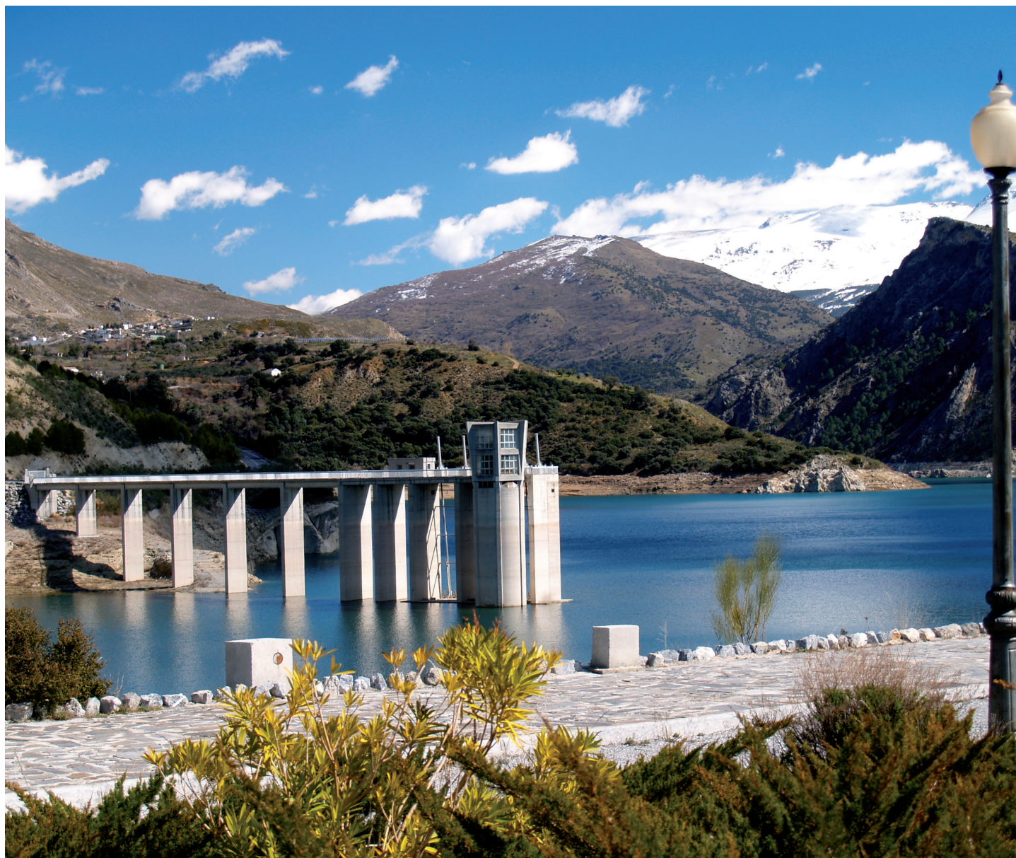
Canales reservoir, river Genil, province of Granada, Spain. The city of Granada drinks water from Sierra Nevada which is regulated at the Canales Reservoir. This reservoir is generated by the Canales Dam, the highest embankment dam in Spain. The water level in the reservoir changes with time, therefore, in order to select the water of best quality, an intake tower has been built, as shown in the picture.
