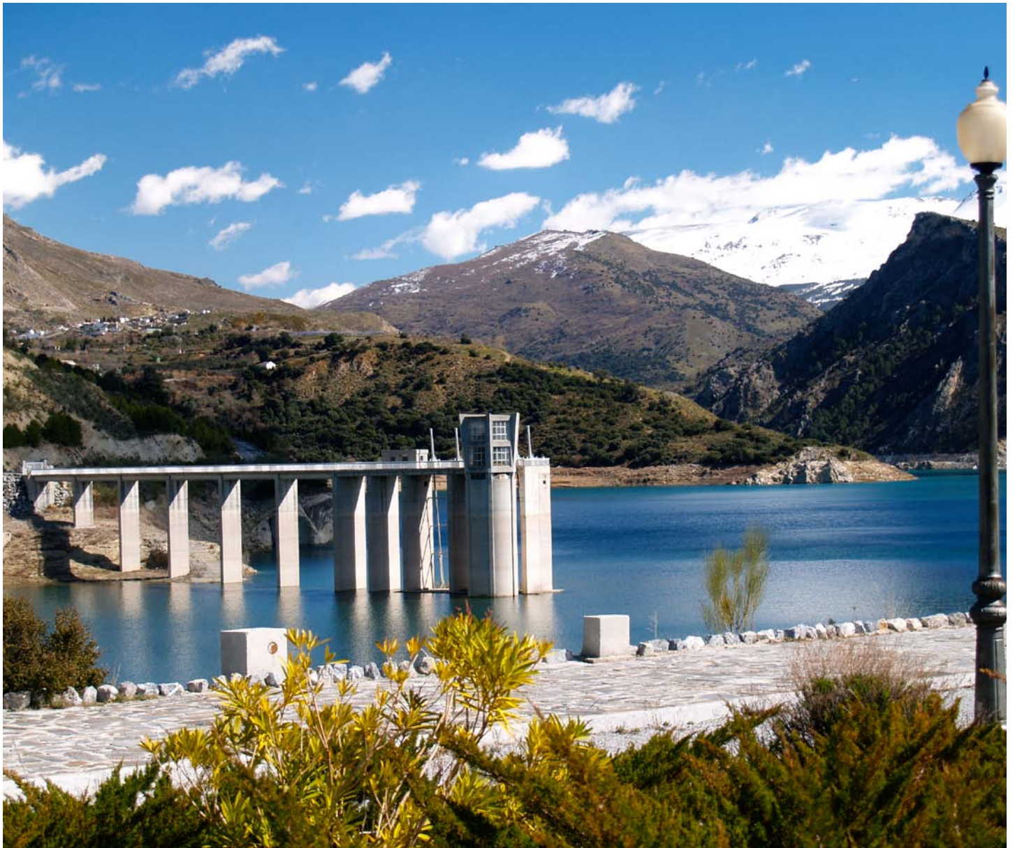
Canales reservoir, river Genil, province of Granada, Spain. The city of Granada drinks water from Sierra Nevada which is regulated at the Canales Reservoir. This reservoir is generated by the Canales Dam, the highest embankment dam in Spain. The water level in the reservoir changes with time, therefore, in order to select the water of best quality, an intake tower has been built, as shown in the picture.
