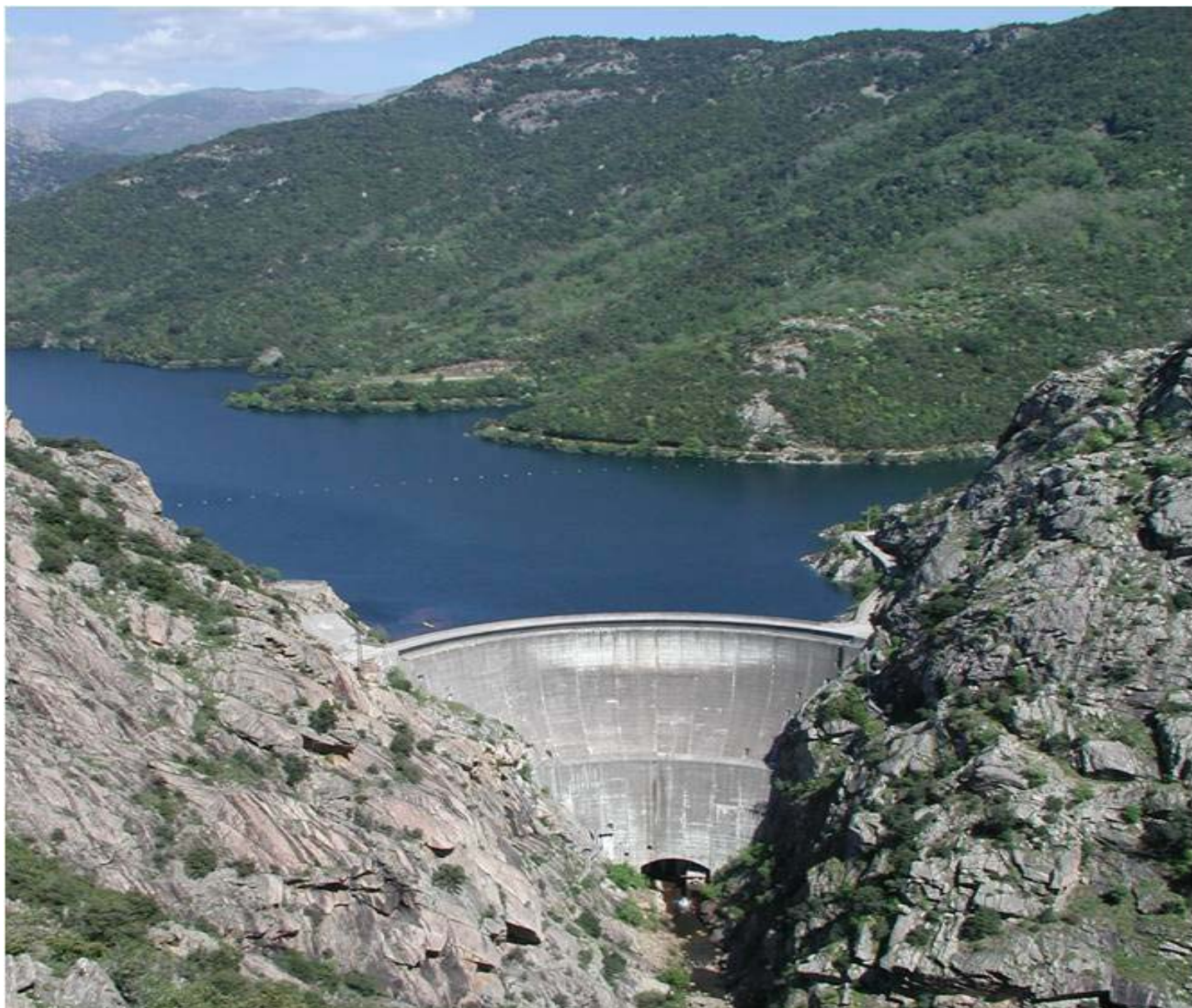
Corsica: Tolla dam - Hydroelectricity and water supply for Ajaccio and its region (South of Corsica). Builded on the Prunelli river in 1960 by EDF, the Tolla dam which contains 31 Mm3 is used for water supply, irrigation and production of hydroelectric energy.
